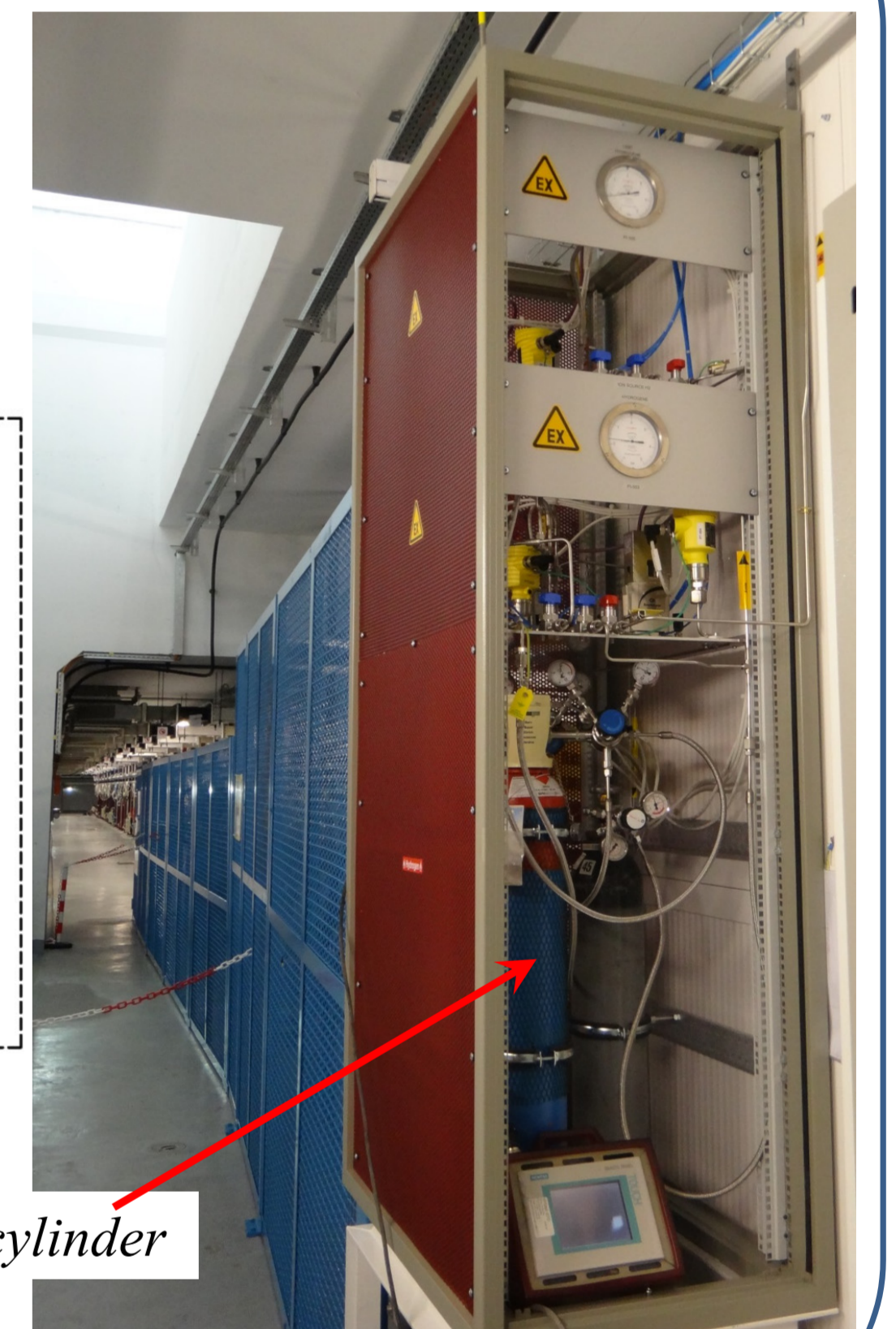
Ion Source and LEBT gas injection rack in the Linac4 tunnel
