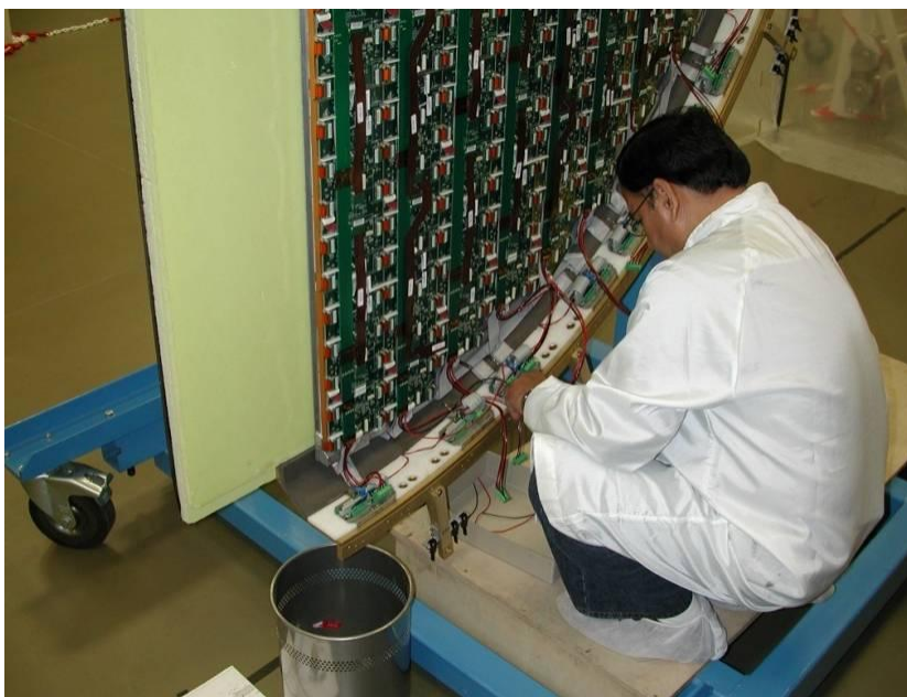
Cabling of the Preshower detector
