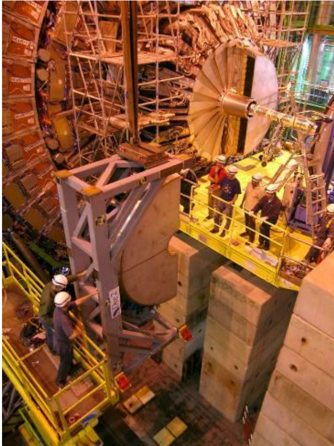
Lifting of DEE 2 on the mounting platform at CMS. DEE 1 is already attached to the HE.
