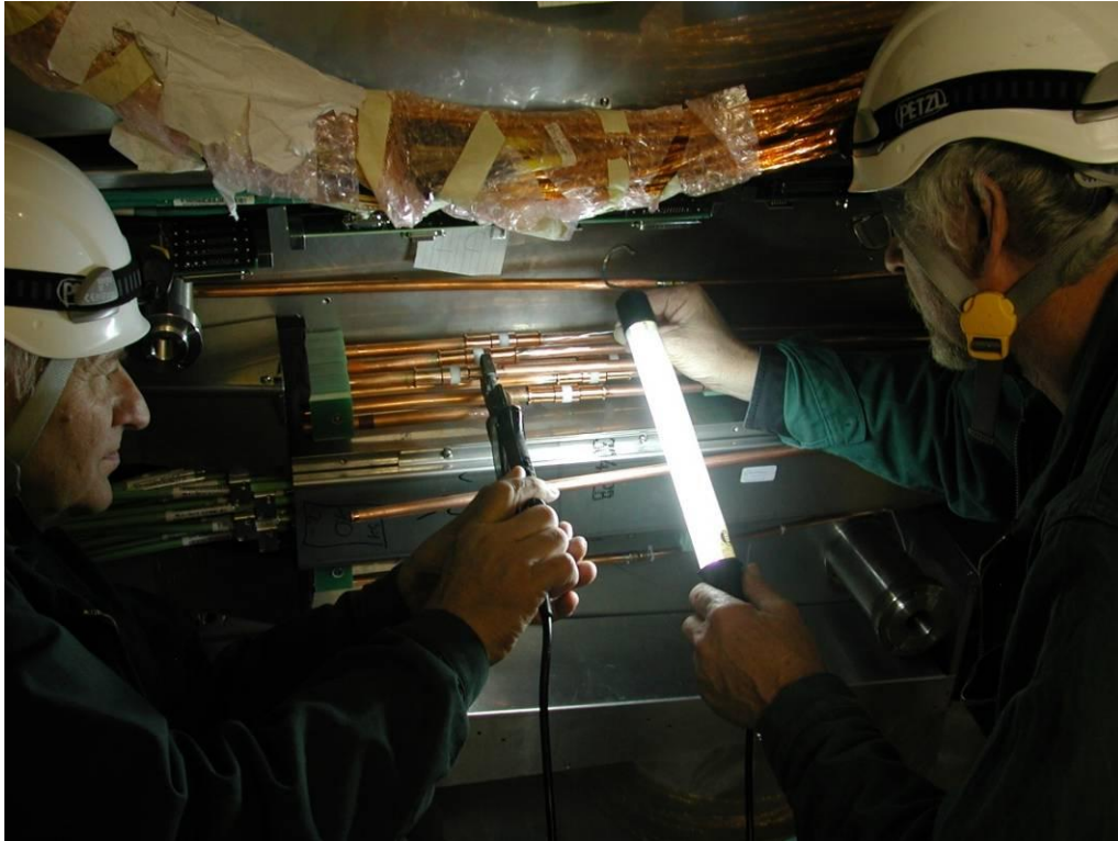
Soldering tracker cooling pipe connections inside the CMS magnet cryostat
