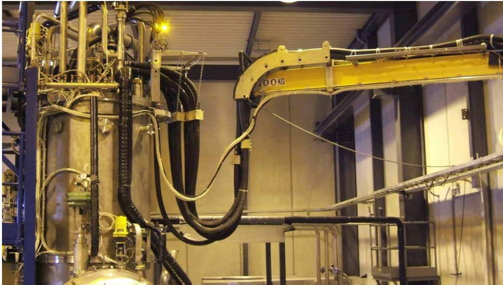
The new support for the magnet power cables
