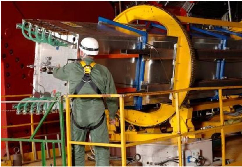
*Photo: Installation of TRD module*
