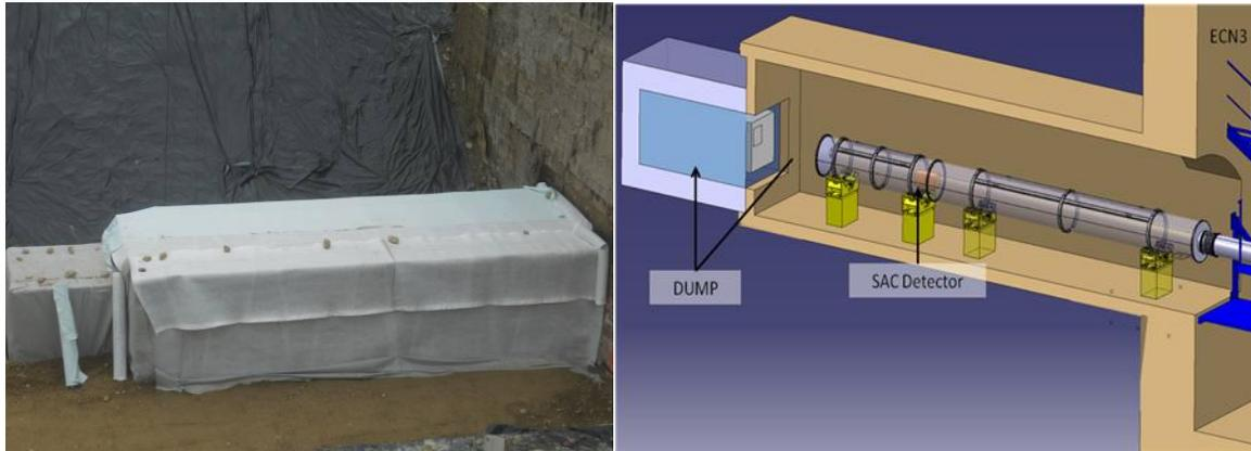
**Photo:** New tunnel and beam dump from outside (left) **3D CAD model image:** new tunnel and beam dump (right)
